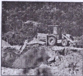
The JCB extracting sand along the Doigrong in Golaghat district.
